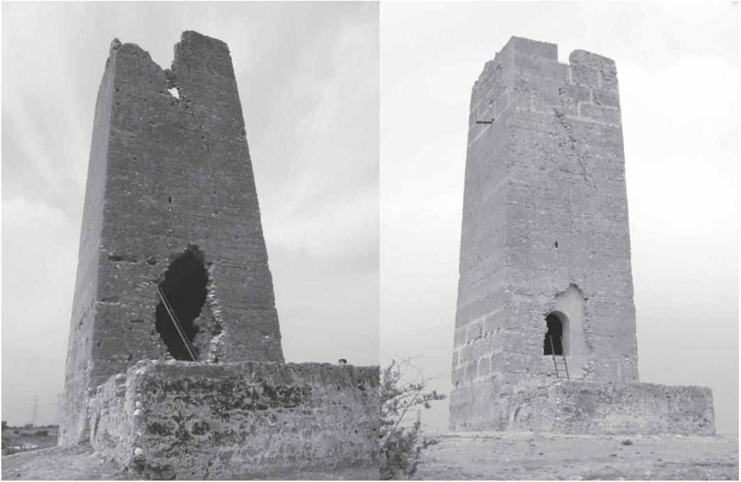
Figure 11. Bofilla Tower before and after the intervention (Vegas & Mileto/Baeza).
