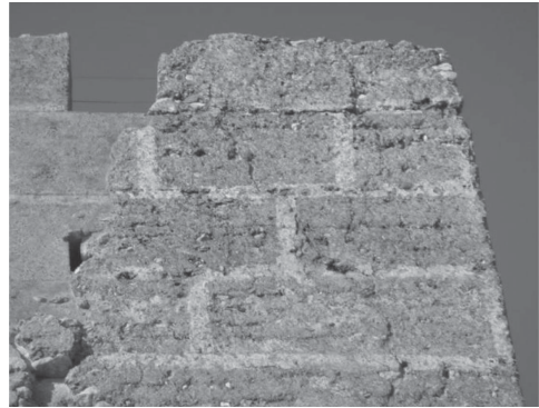
Figure 9. Tower crown with consolidation and reintegration treatments (Vegas & Mileto).
